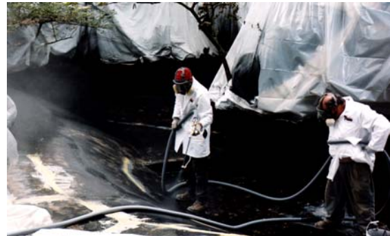
Low-Pressure Polyurea Being Utilized on Concrete as a Fish Pond Liner
