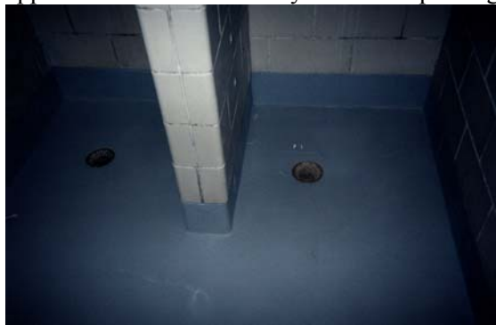
Roadside rest areas, such as this one in Texas, are a perfect size application for low-pressure applied polyurea
