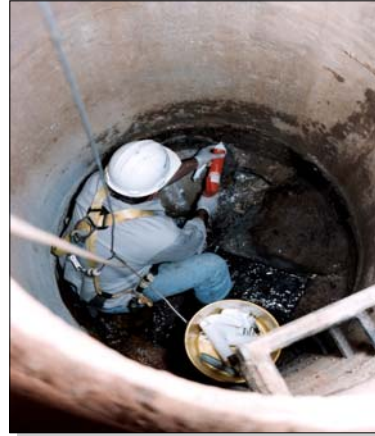
Mike Kronz of ROI installing Hydraloc Extreme
