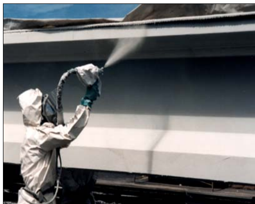
Spraying the girders on the San Mateo Bridge Project
