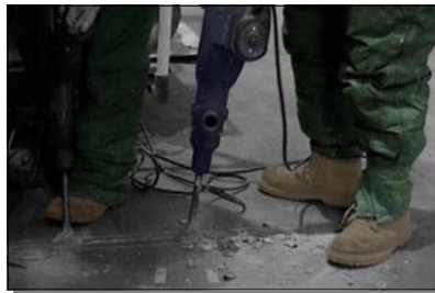
Above pictures: Concrete surface prep in -26°F temperature.
