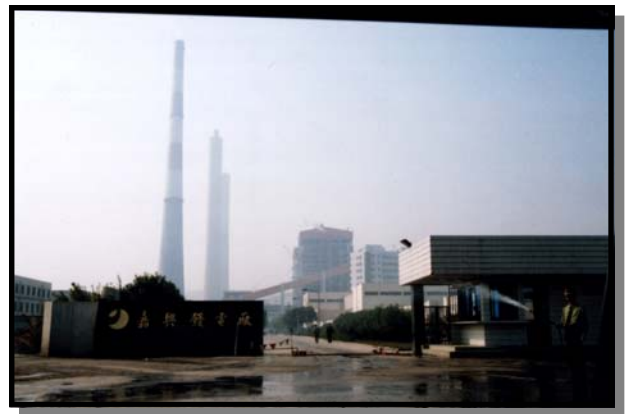
Jiaxing Power Plant South of Shanghai, China
