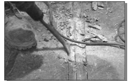
Above pictures: Concrete surface prep in -26°F temperature.
