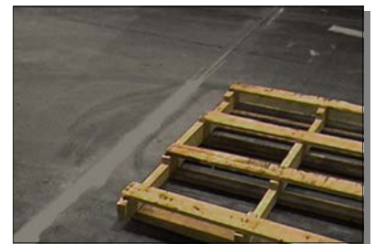
Picture after installation of ES-2350 polyurea
