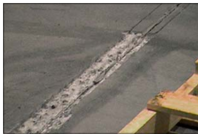
Picture of joint after it has been prepped
